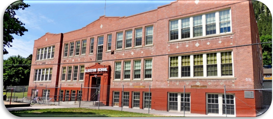
Image 15: Alberton School - Credit Jeff Crews
